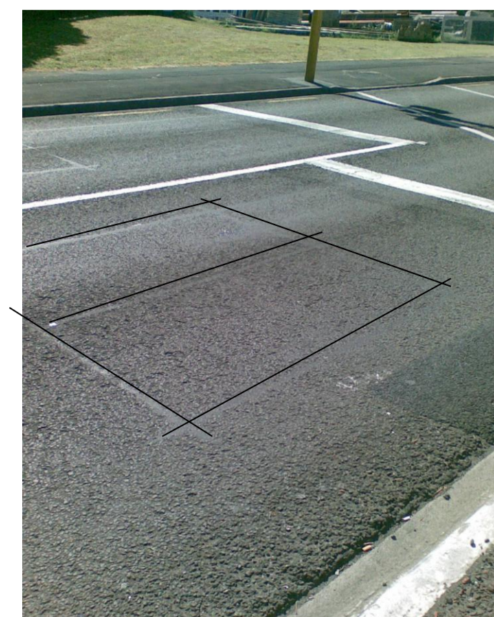
Stop Line Vehicle Detectors
